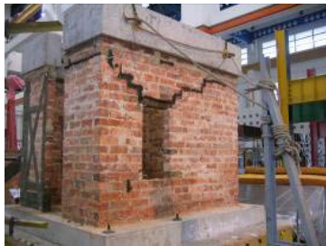
(a) PGA = 0.30 g: Cracks at upper portion
